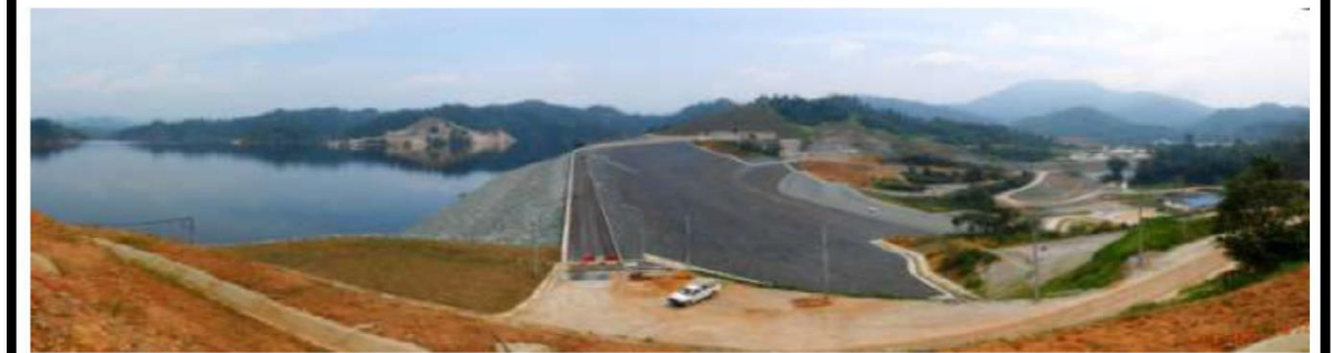
Overview of Puah Dam and Lake from Right Abutment
