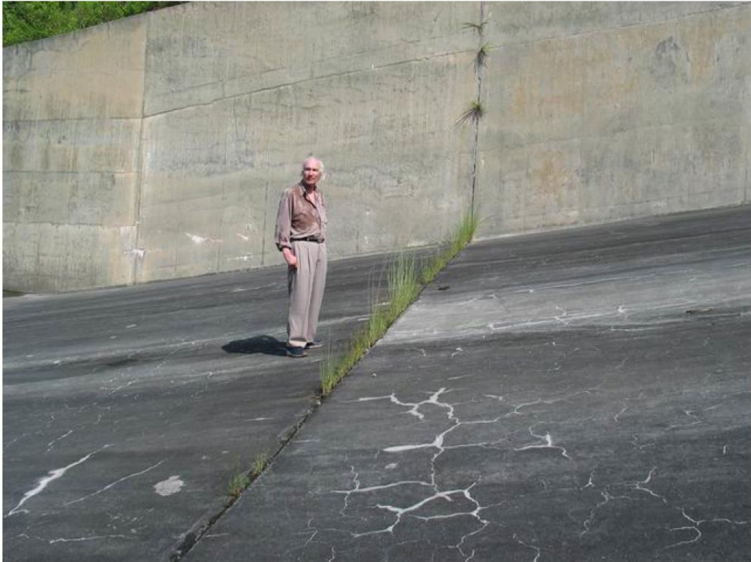
Picture T5 – Spillway Joints
