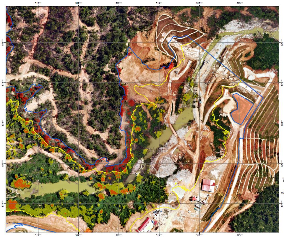
Lidar view of Tembat dam during construction. Yellow line indicates reservoir FSL.
