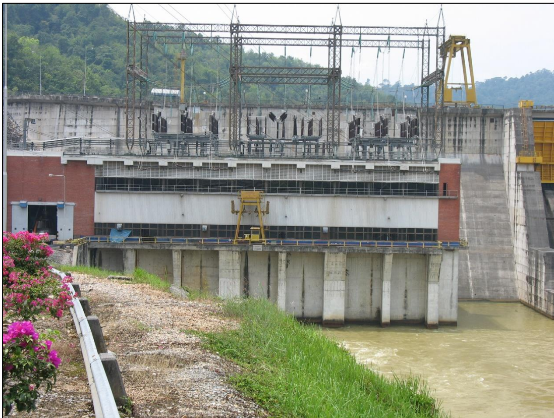
Kenering Powerhouse view 2006
