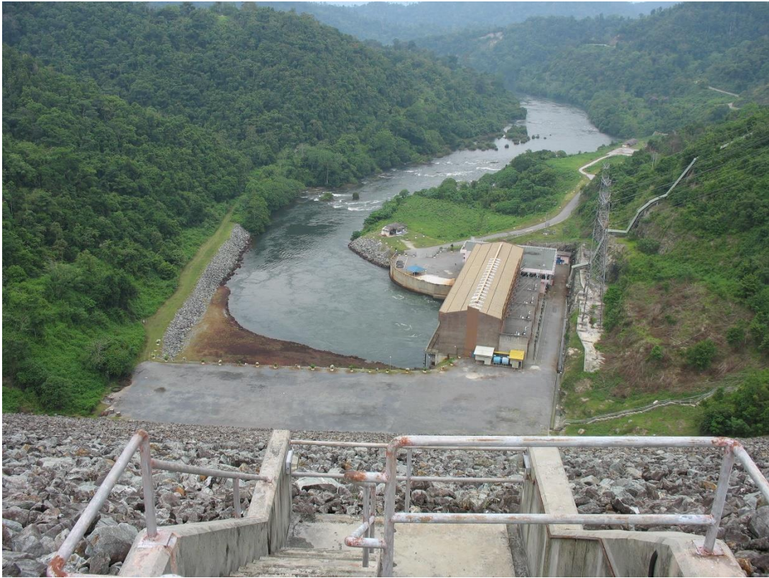
Temengor Powerhouse viewed from dam top
