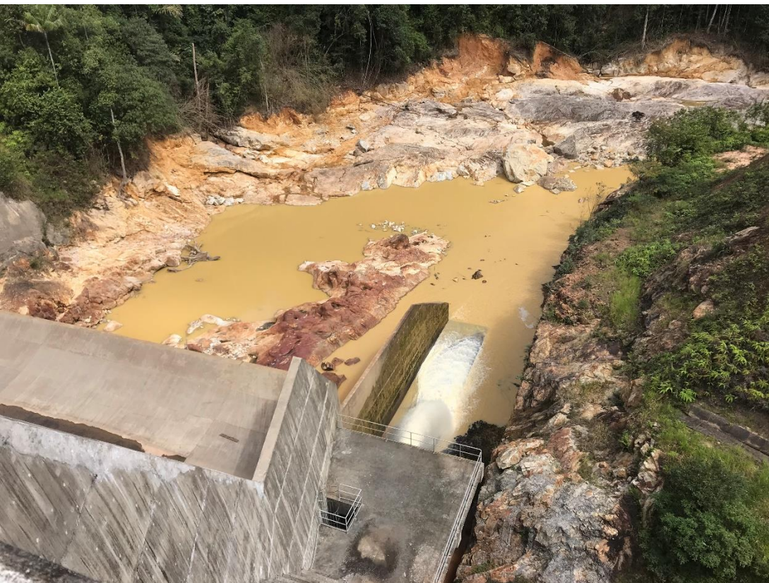
Rocky riverbed after spilling during 2019 NE monsoon. 0.5 m 3 /s riparian release January 2020
