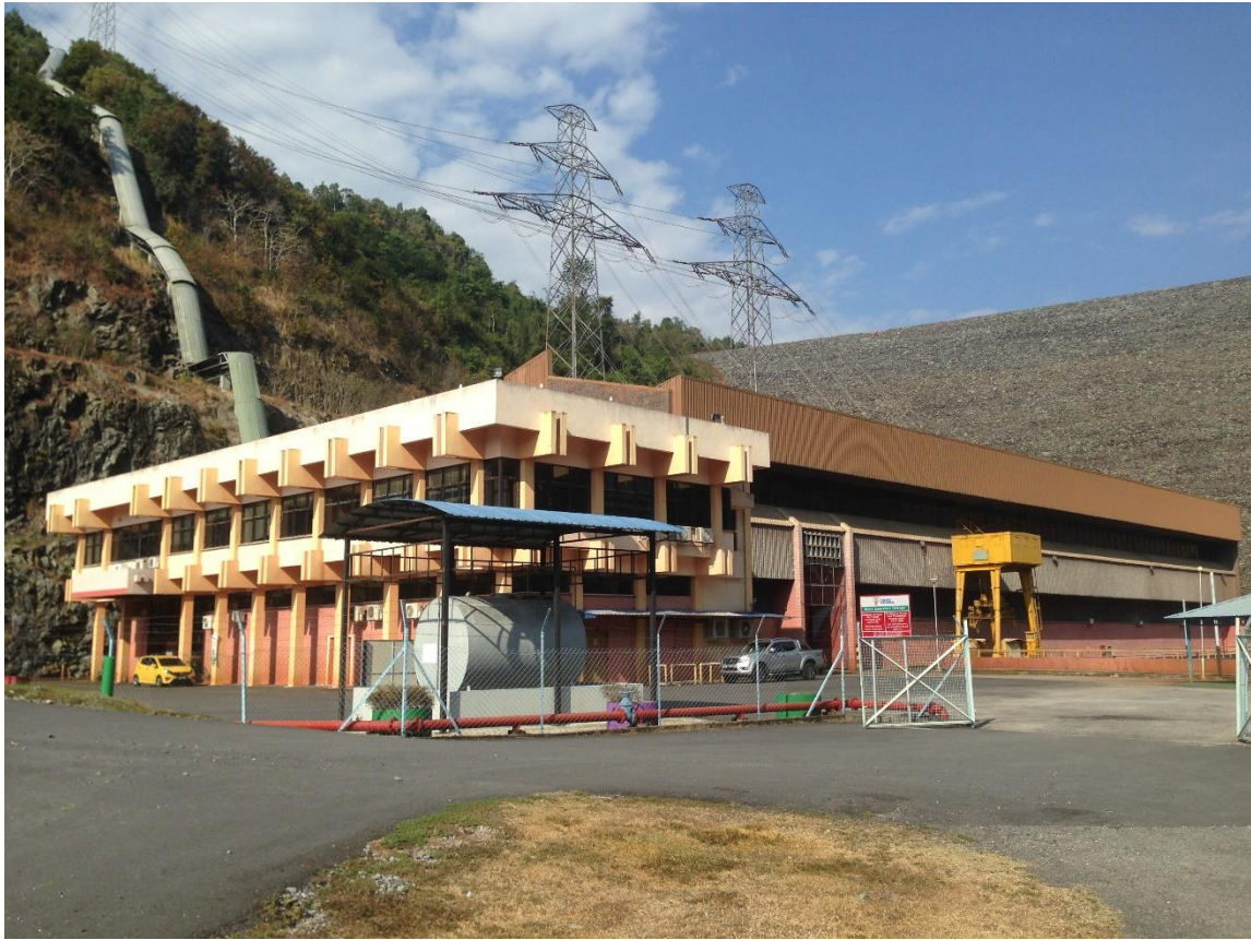
Powerhouse viewed in January 2020.
