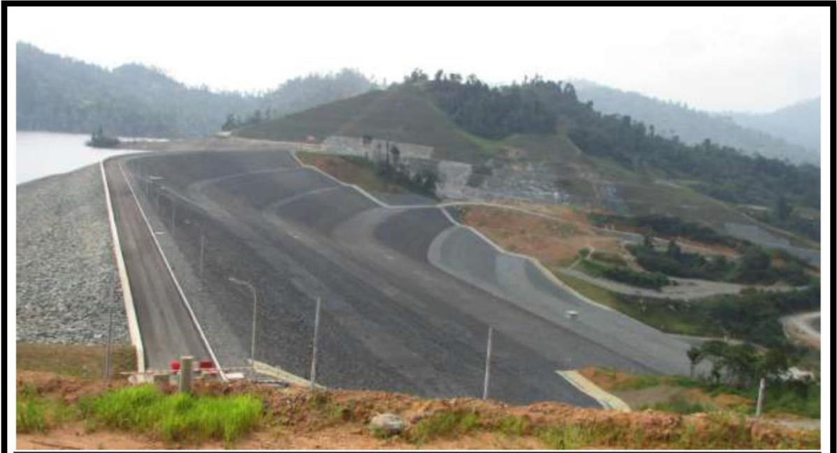
Puah Dam viewed from Right abutment.
