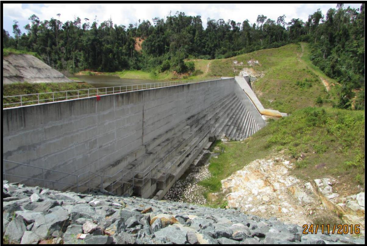
Tembat Dam viewed from Right Bank
