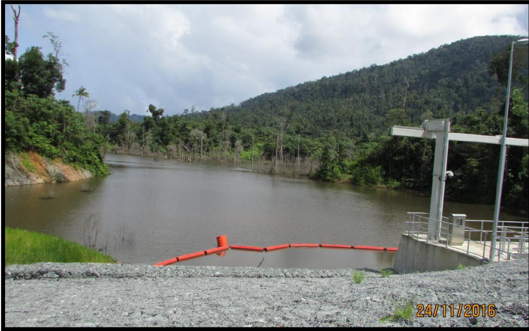
Tembat Intake Forebay and Logboom
