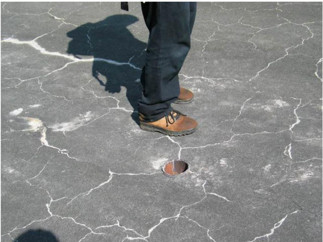
Picture T12 – Spillway Chute
