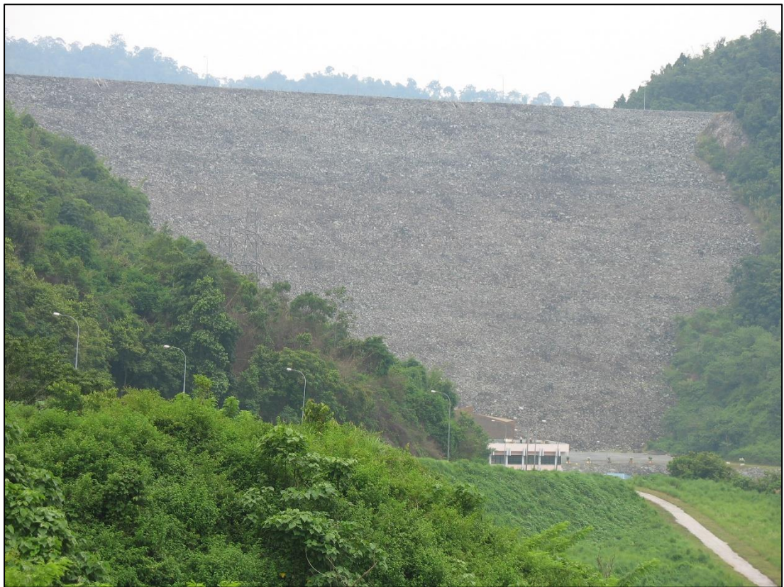
And dam viewed from below; powerhouse in lower foreground.
