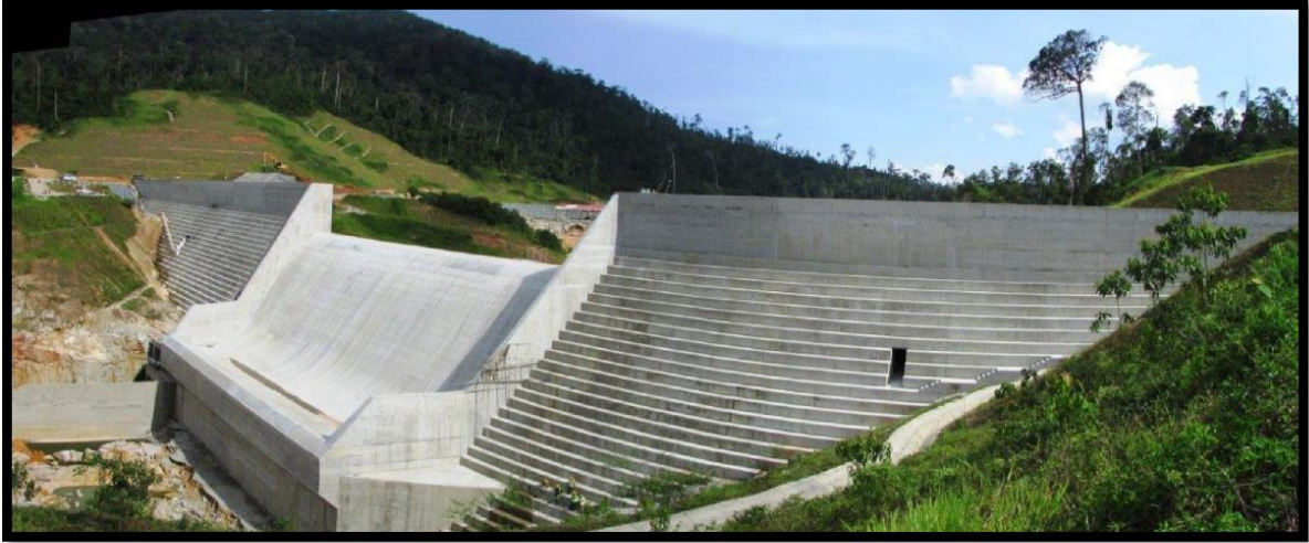
Tembat Dam viewed from Left Bank
