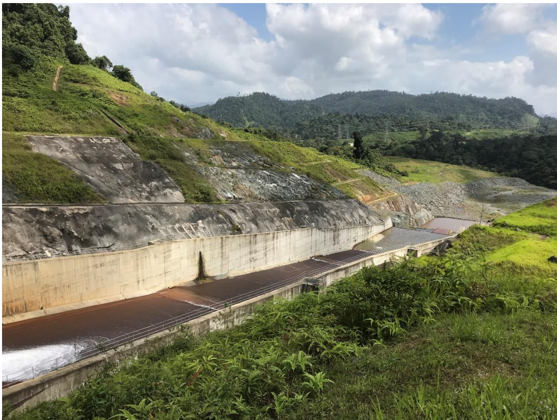
And downstream view. 275 kV Transmission line LIL connection in background
