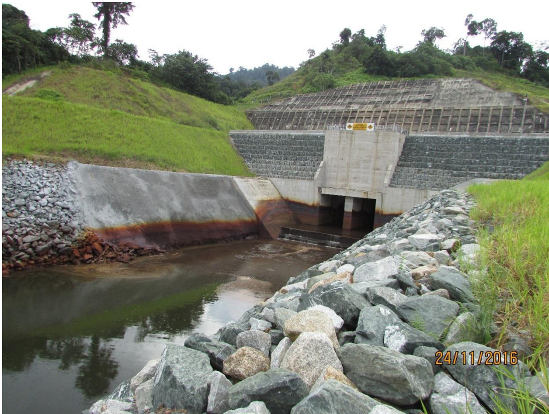
Tailrace outlet as completed with Gabion Weir.
