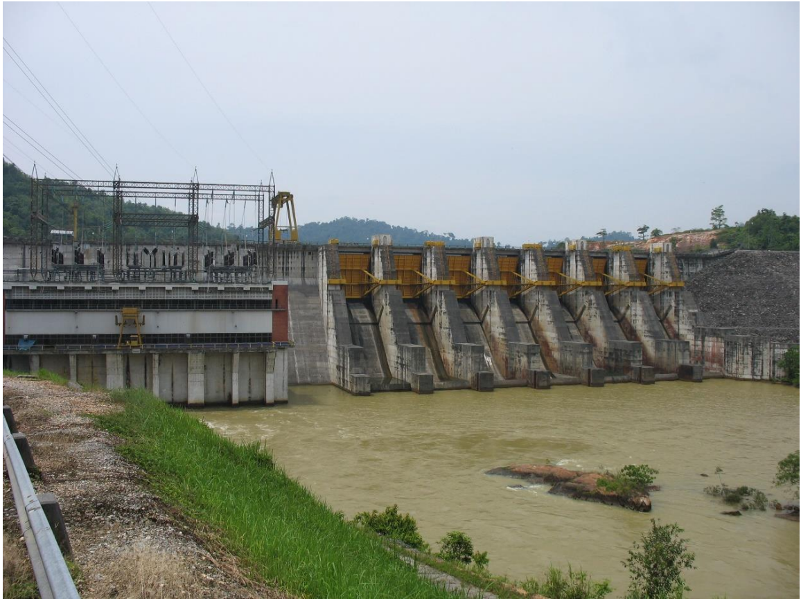
Kenering powerhouse and spillway 2006.
