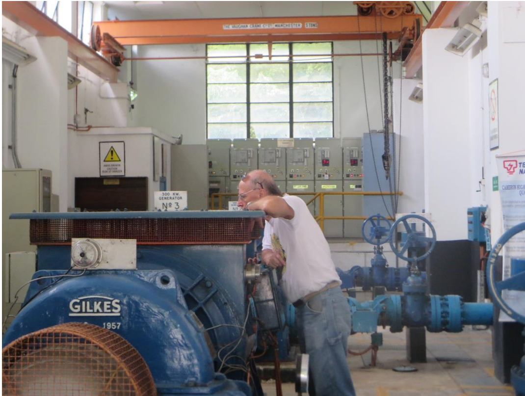
Impromptu inspection of the 1957 Robinson Falls Turbine by a curious Electrical Engineer
