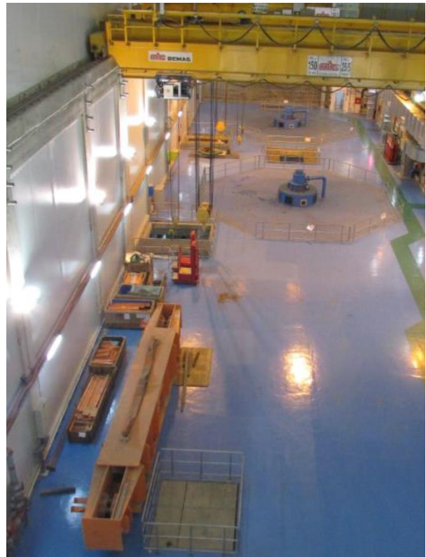
Puah 2-unit Power cavern completed with Giertsen PVC drip ceiling.
