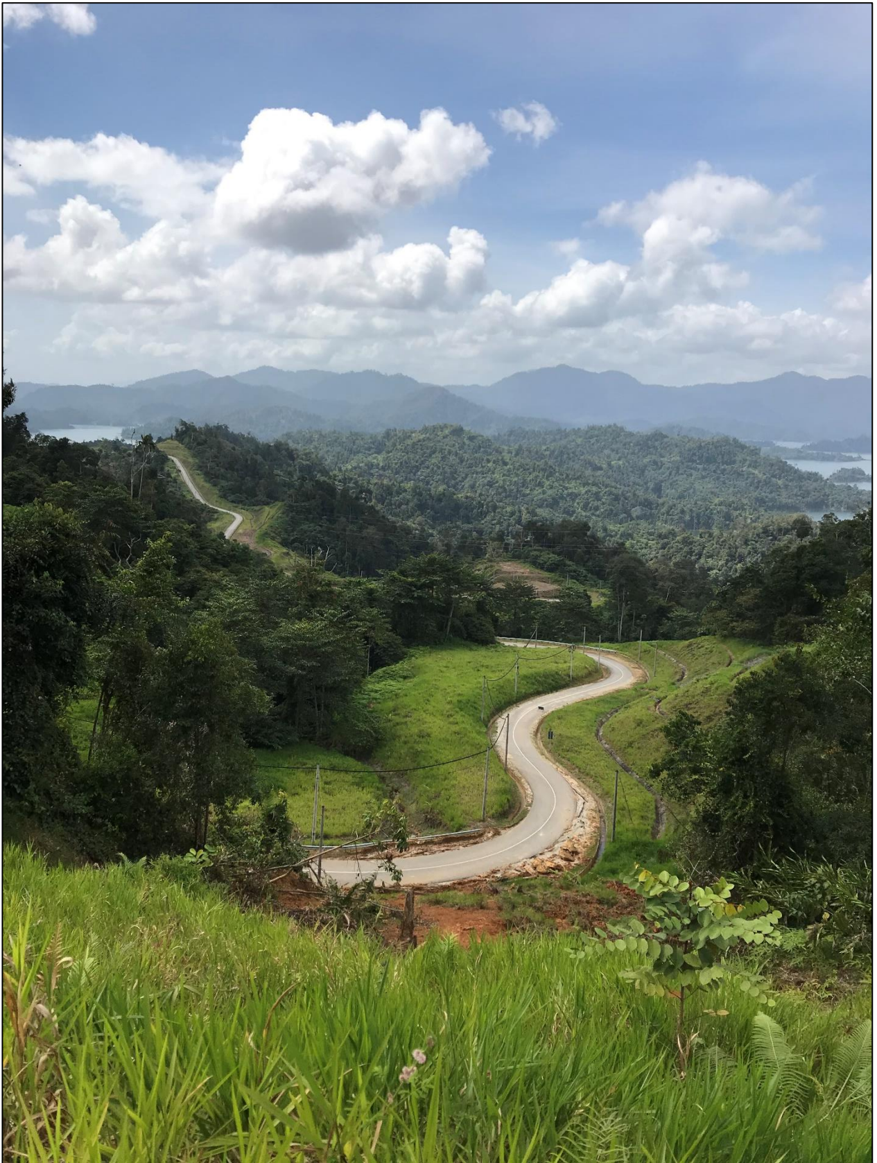
The winding 10 km road to Tembat with Puah Lake in background January 2020
