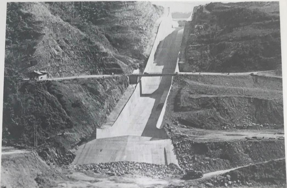
#58 Spillway — View of Completed Chute and Flip Bucket — 28 April 1978
