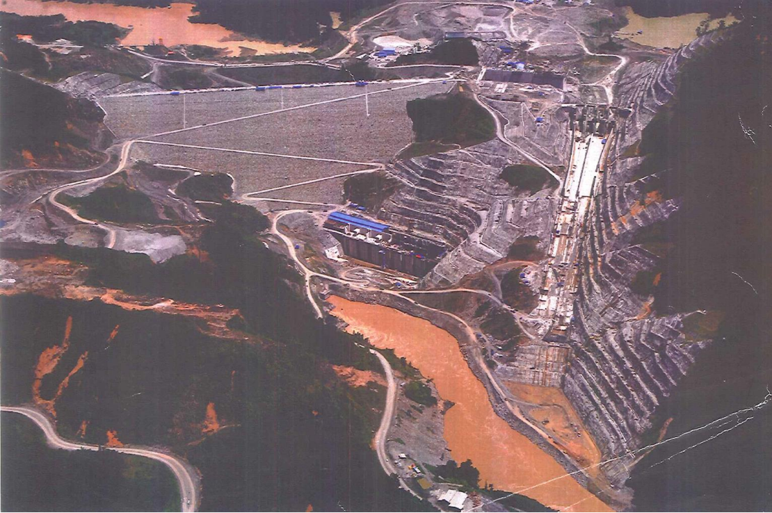
Spillway under construction.....
