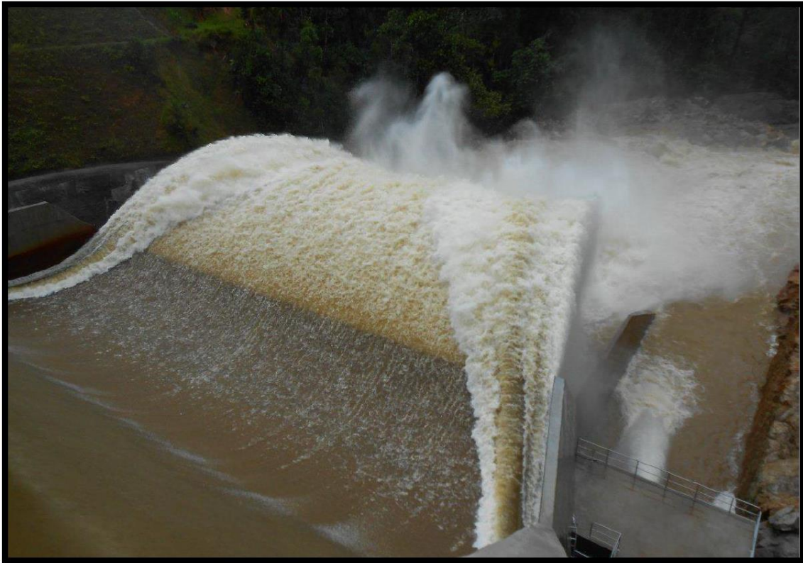
Tembat Spilling – Tapered chute from 60m to 40m. Riparian release a bottom right
