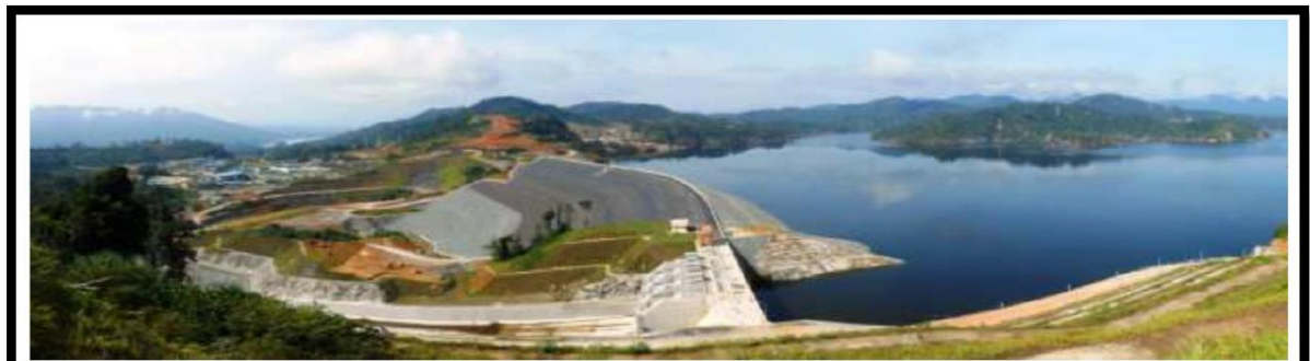
Overview of Puah Dam, Spillway and Lake from Left Abutment
