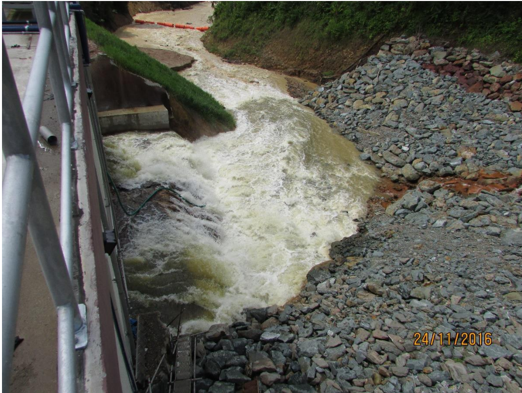
Tembat Tailrace outlet to Puah Lake.
