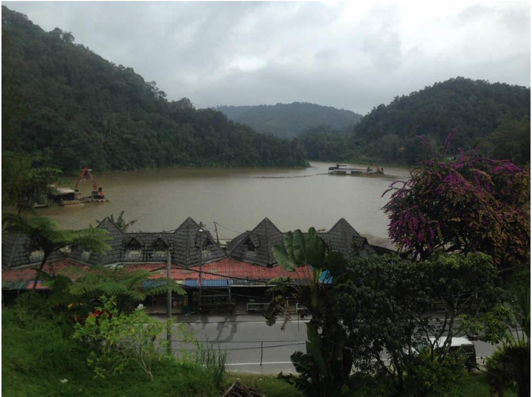
Ringlet Lake dredging using Backhoes on pontoons in 2019.
