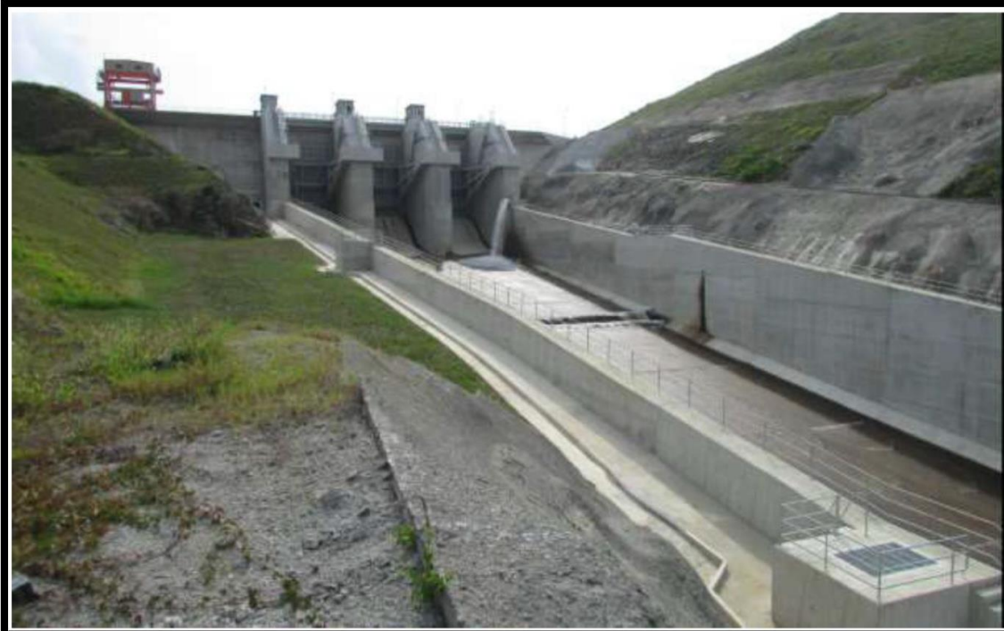
Puah Spillway looking Upstream
