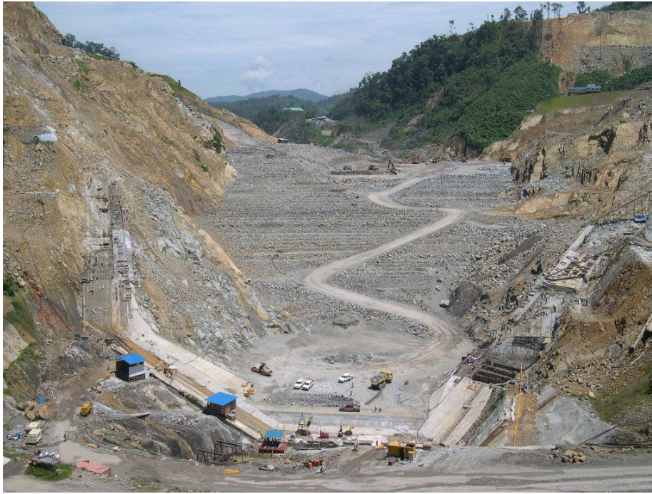
View of plinth construction
