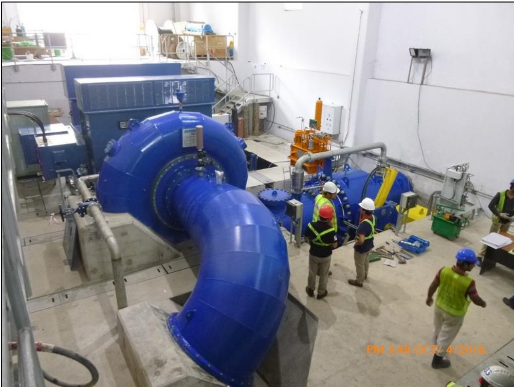
Tembat Powerhouse: 2 x 7.5 MW horizontal axis Francis units, installed after refurbished by REMACO
