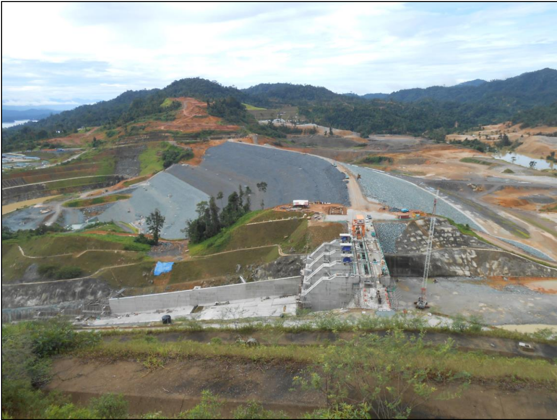
Puah Spillway and Dam during construction.
