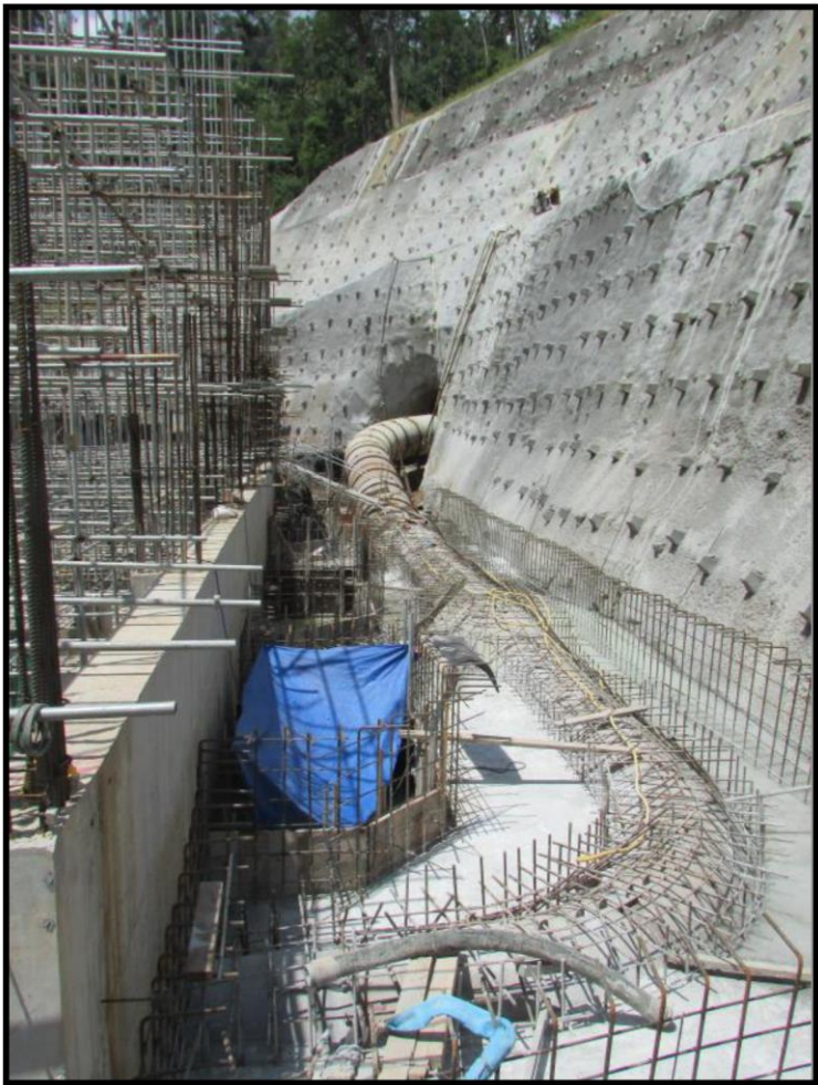
Tembat Powerhouse Manifold during Concrete surround placement
