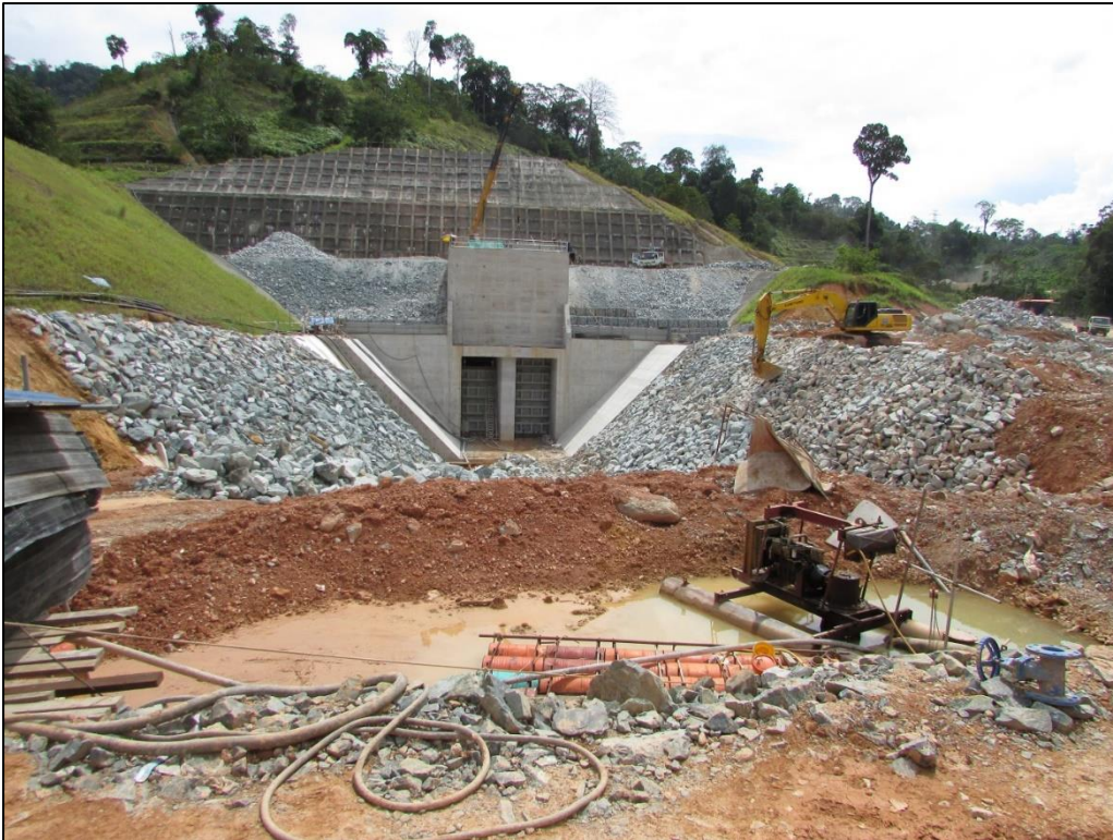
Puah Tailrace outlet gate structure during construction
