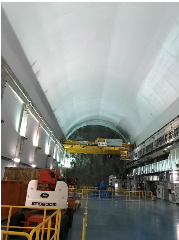
Puah 2-unit Power cavern completed with Giertsen PVC drip ceiling.
