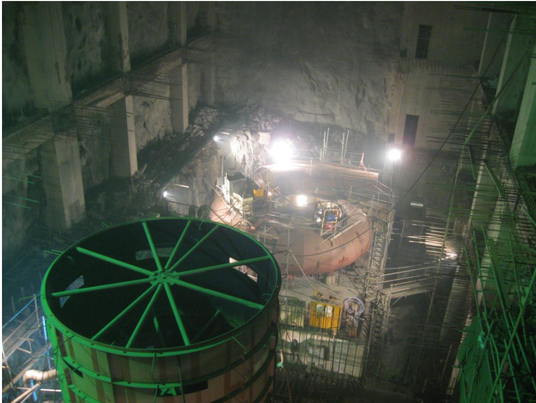
Puah Underground powerhouse during spiral case Installation.
