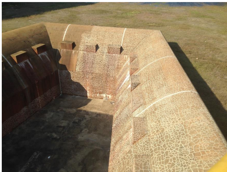
Repairs to surface crest cracks, January 2020 photo.
