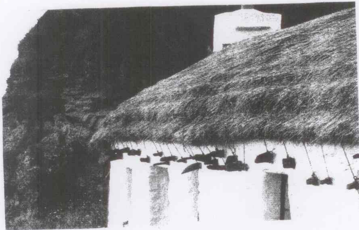
Tying down a thatched roof
